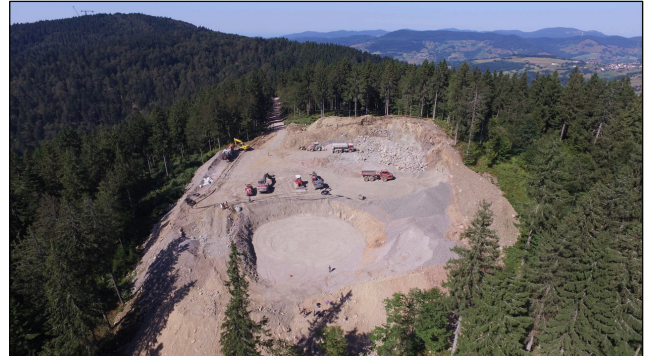
Windfarm Gersbach in the Black Forest (Germany), 2023 under construction. (Picture Freie Landschaft Schweiz)
